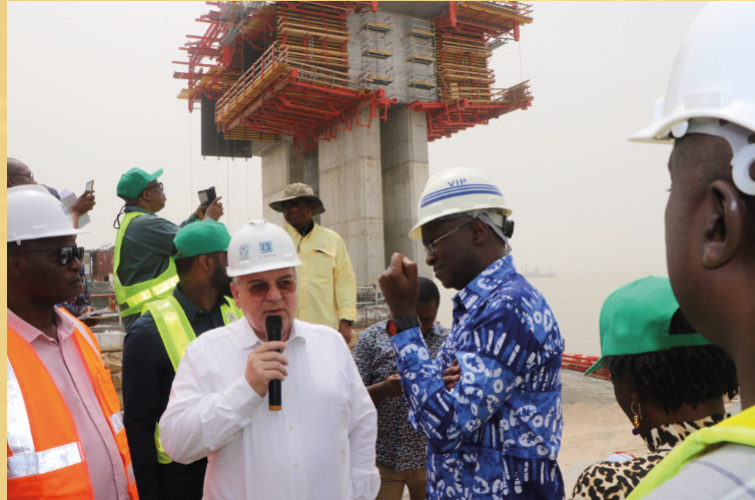
Hon Minister Babatunder Fashola SAN (right) being briefed by the Project Director, Engr. Friedrich Josef Wieder (middle) during the inspection of the 2nd Niger bridge in Anambra and Delta States, 11 February 2020
