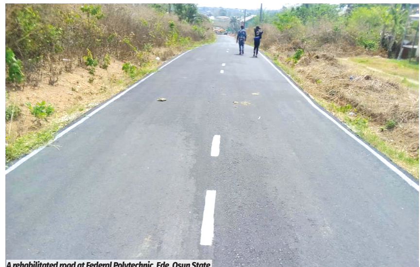
A rehabilitated road at Federal Polytechnic, Ede, Osun State
