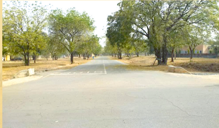
A newly rehabilitated road at Bayero University, Kano, Kano State
