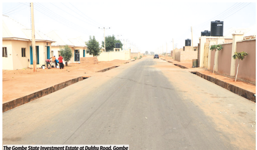
The Gombe State Investment Estate at Dukku Road, Gombe
