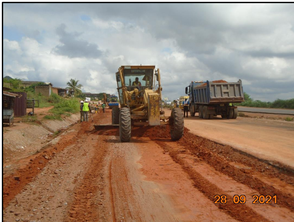
EXCAVATION OF EXISTING FAILED SHOULDER BETWEEN CH 26+000 AND CH 26+210 (LAGOS BOUND)
