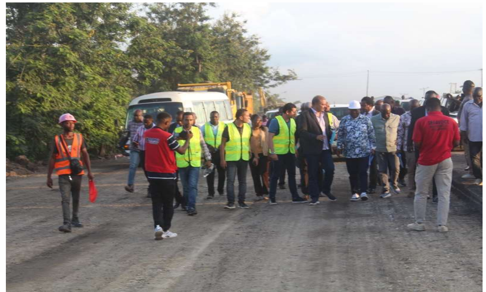
REHABILITATION OF IBADAN-OYO DUAL CARRIAGEWAY IN OYO STATE, KM0=000 - KM 43=000, ROUTE NO. 20(A1)WR.16222/I C/NO7644
