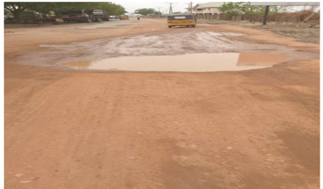
YOLA-HONG-MUBI ROAD IN ADAMAWA STATE, NORTH EAST
