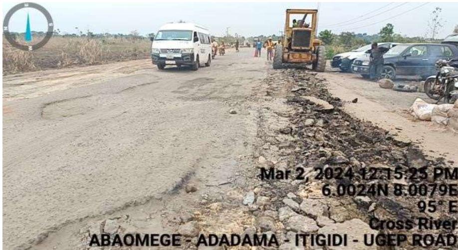
BEFORE (CH.0+00 – CH.0+200)
