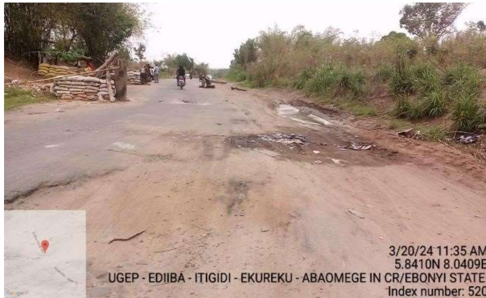
ONGOING (CH.0+200 – CH.0+650)
