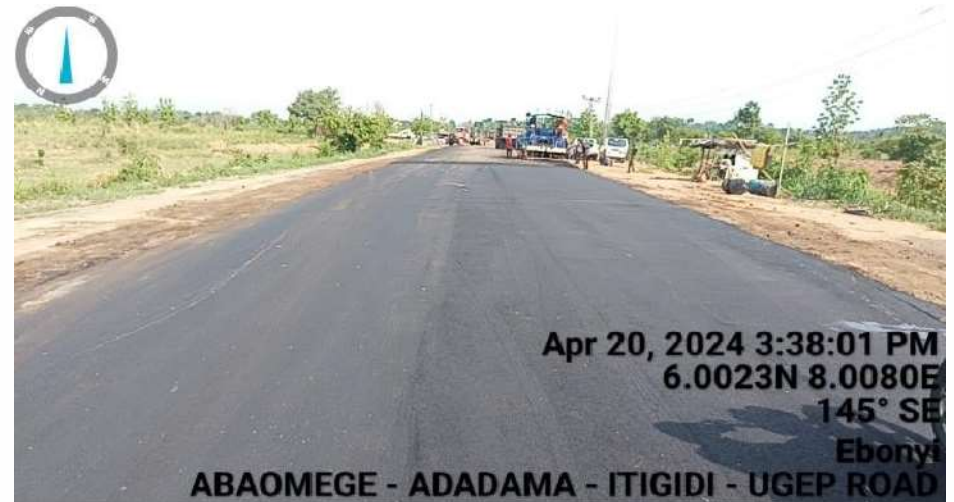
ONGOING (CH.0+000 – CH.0+200)
