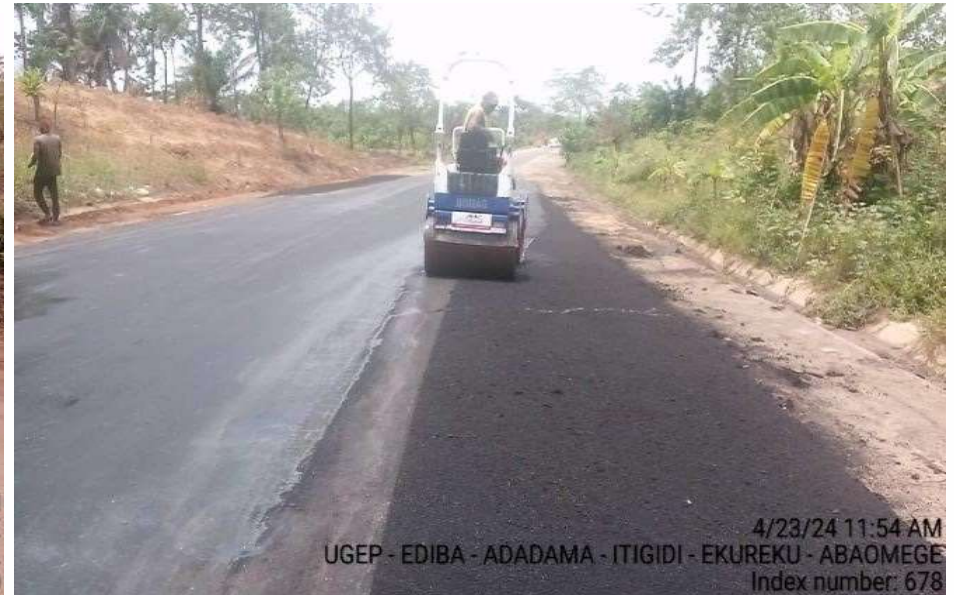
ONGOING (CH.0+000 – CH.0+200)
