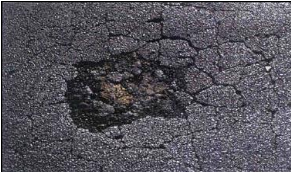
Figure 20: Pothole Developing
