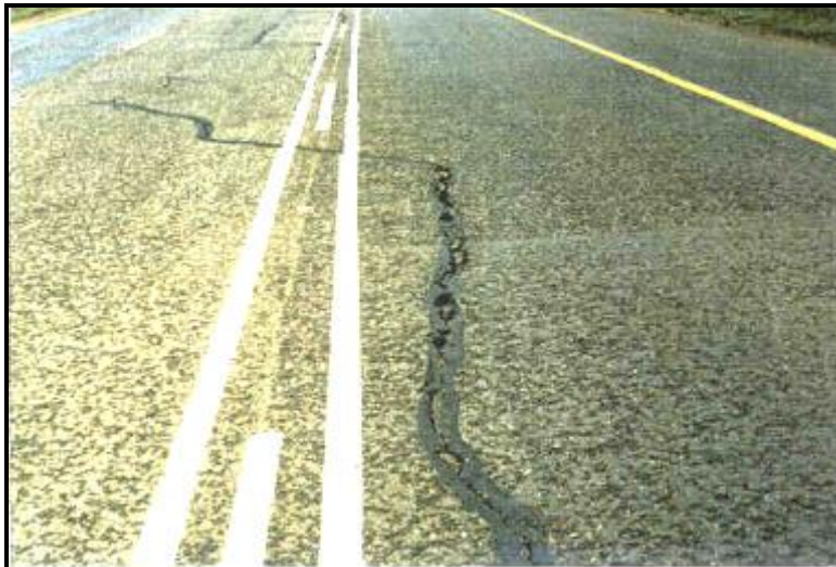
Figure 26: Slippage Cracks
